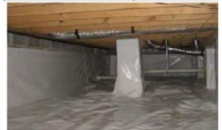
**NOTE:** Completely sealed crawlspaces (no exterior cross-ventilation) require a dehumidification system as part of the sealed crawlspace design.
